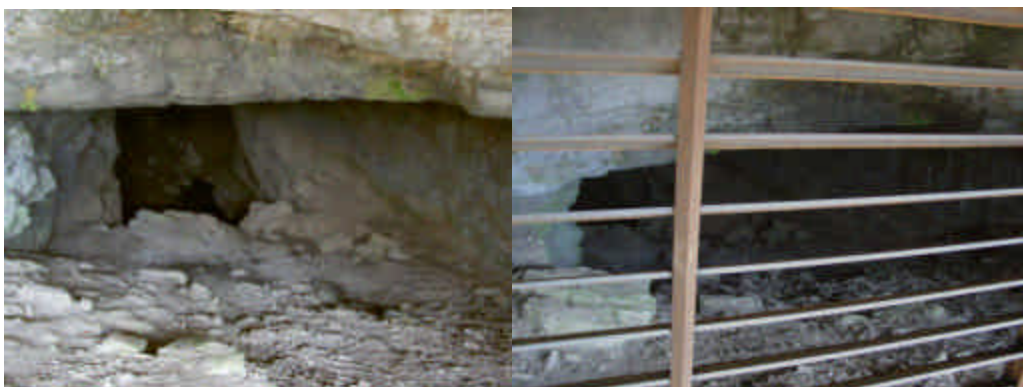
Figure 2. View into Owl Cave on left. Graffiti on exposed ledges and artifact pilfering necessitated a gate. Impact to pretty sunbeams entering the cave was minimized by angling flat bars like venetian blinds. No bat use had been previously documented.
